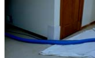
Corner guards and drop clothes are routinely used to protect your home.
